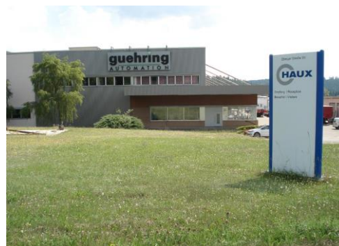
Plant in Stetten a.k.M. - Germany
